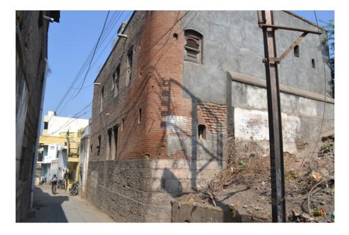
Traditional courtyard houses in the western part of India, particularly Maharashtra, known as wadas are built in local stone or brick in lime mortar and a structural wooden frame consisting of teak columns and beams that act as tie members for the structure.
