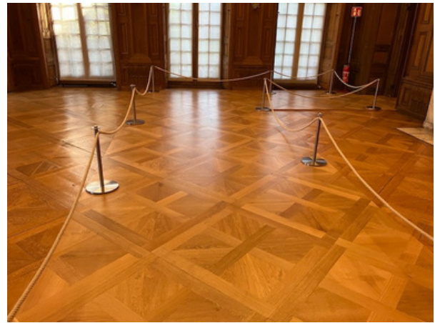
Fig. 5 A nice example of the protection of a historic parquet floor: Newly laid parquet over the historically preserved floor
