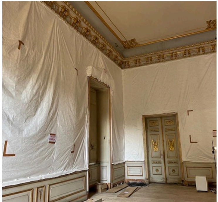
Fig. 10 Preconstructed "boxes" as dust protection
