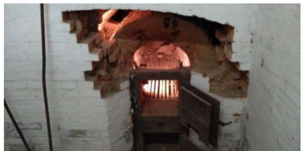
Historic warm-air-channel-encased-flue-heating system at the orangery wings of the Orangery Palace
